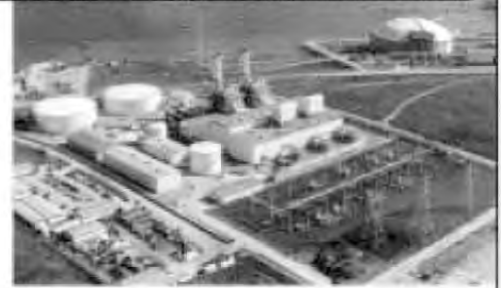
478 MW MARMARA NATURAL GAS COMBINED CYCLE POWER PLANT, TURKEY
